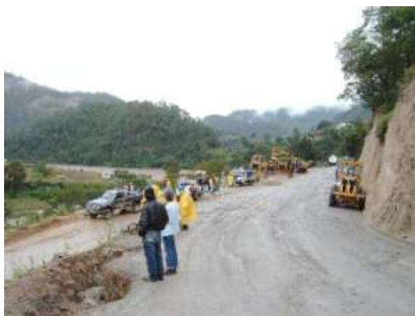
Reconstruction of basic infrastructure after hurricane Stan.
