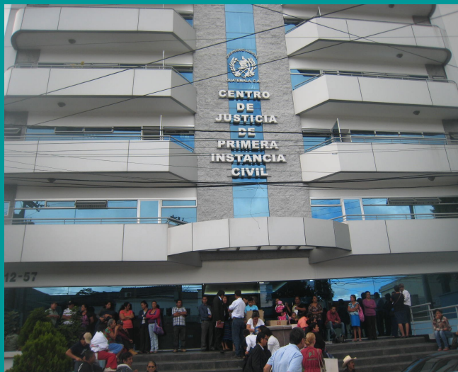
Hearing to resolve an appeal against the construction licence for El Tambor mine. 6 July. Photo: PBI
